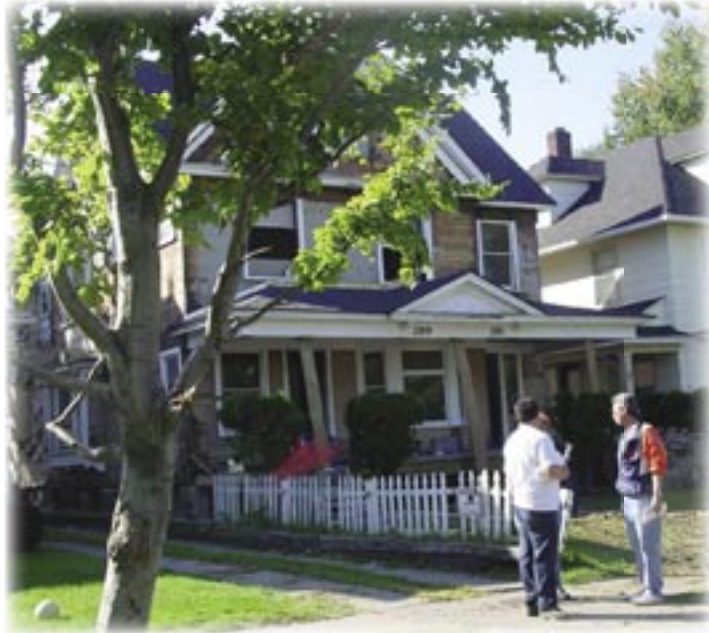
Northern Star contractor Michael Spaan and Greater Rochester Housing Partnership Rehab Specialist Steve Davis discuss rehab of Lakeview double.
