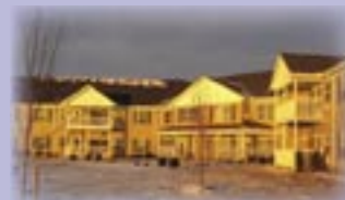
Union Park, North Chili, an affordable senior rental community, received its Certificate of Occupancy in December 2004.
